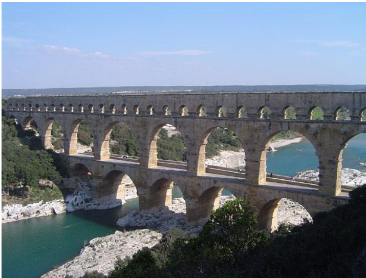
Figure 1 - “Pont du Gard” aqueduct, built in France during the 1st century with lime/pozzolan mortars.
