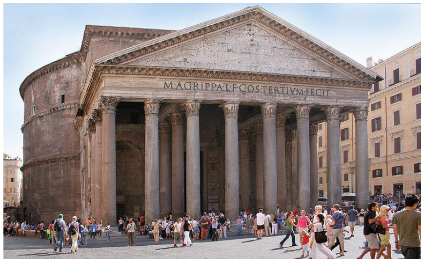
Figure 2 - Pantheon, built in Rome during the 2nd century. The perfect semi-circular rotunda was realized with lime/pozzolan concrete with different density from bottom to the top, in order to reduce tensile stresses.
